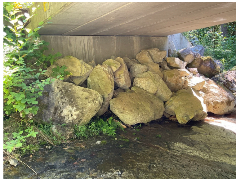
Left Bank Abutment when facing downstream
