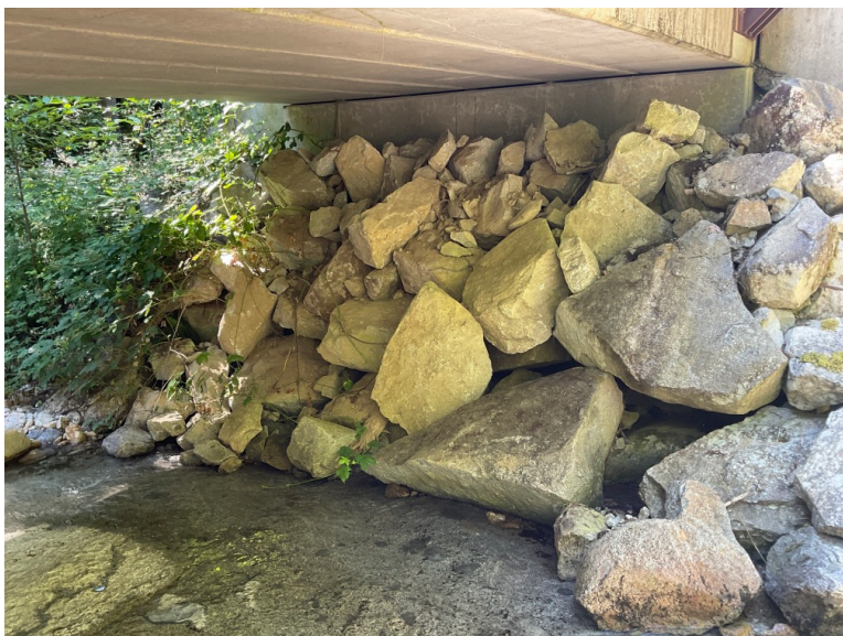
Right Bank Abutment when facing downstream
